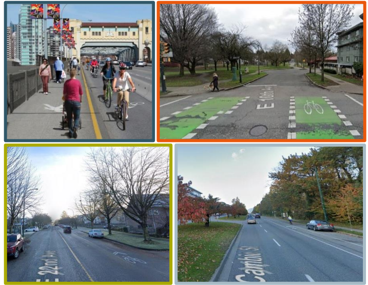
Examples of each type of infrastructure from top left clockwise: protected bike lane on Burrard Bridge, local street bikeway on E 10th, painted lanes on Cambie St, and shared bike lanes E 22 nd Ave. Credit Google maps
